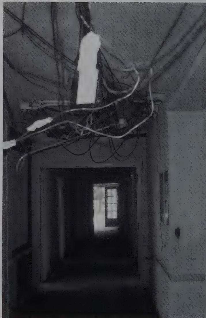
A new, more efficient, less costly lighting system, equipped with better backup has replace Sewell's old one. Photo by Kylie Beck.
