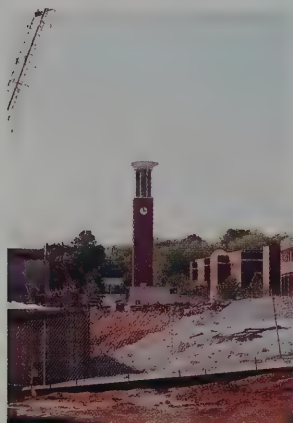
Right : The Belltower rises above the excavation for the new arena.
